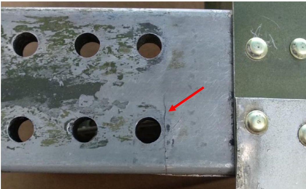
Figure 7. Example of Cracks Not Intersecting Outboard Bolt Hole PA-28-181, 12,824 hours TIS
